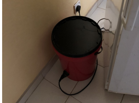
A portable hot water tank that plugs directly into 240 volt power
