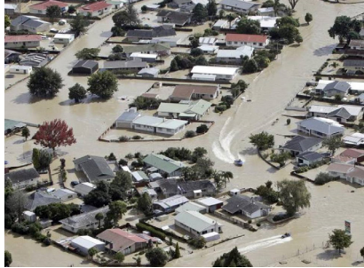
Rangataiki River Stop Banks Broke and the town of Edgumbe was flooded
